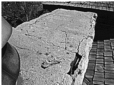
Damaged Chimney Cap
