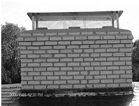
Metal Cap on Clay Liner Chimney Top
